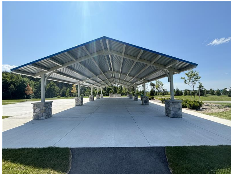
New shade structure at Henderson Park
