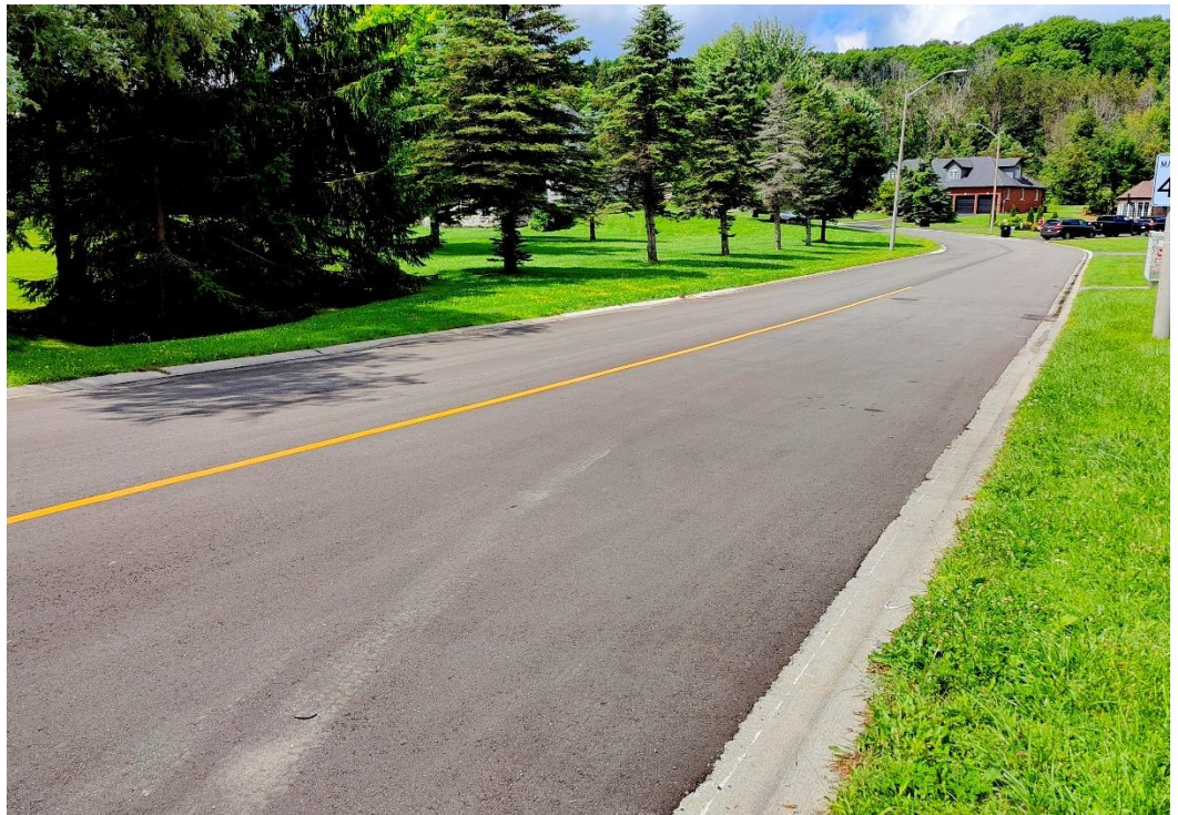
The newly repaved Kilkenny Trail
