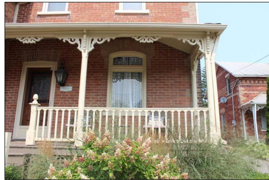
4334 County Rd. 88 – front porch (Source: GDV)
