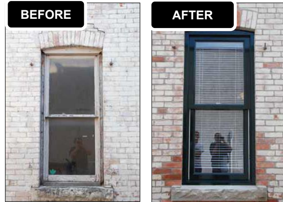
Example of window and exterior façade restoration / replacement based on historic documentation of originals. (Source: Standards and Guidelines)
