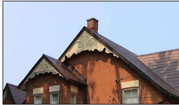
2870 County Rd. 27 – Gable details (Source: GDV)
