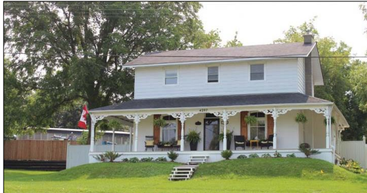
4297 County Rd. 88 – Wrapping verandah (Source: GDV)
