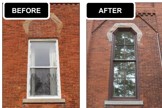
Example of window restoration / replacement based on historic document of originals. (Source: GDV)
