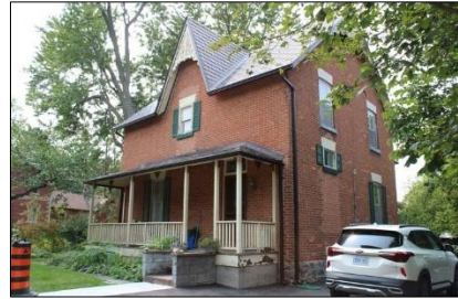
2870 County Rd. 27 – Front porch (Source: GDV)
