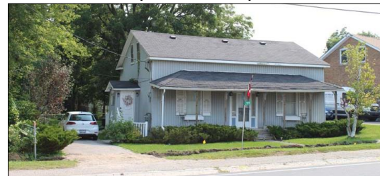
2891 County Rd. 27- Front porch (Source: GDV)
