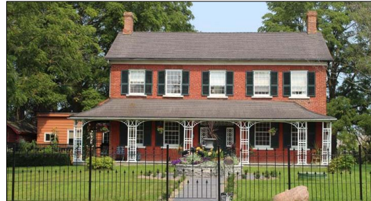
4370 Line 7 – Verandah (Source: GDV)
