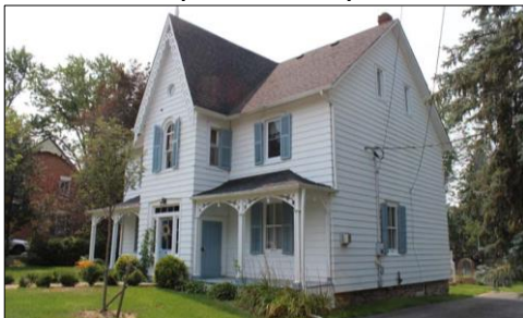
2876 County Rd. 27 – Front porches (Source: GDV)
