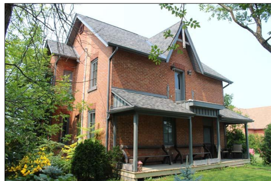
62 Hearn St. – front porch and former upper balcony (Source: GDV)
