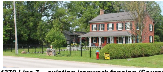
4370 Line 7 – existing ironwork fencing (Source: GDV)
