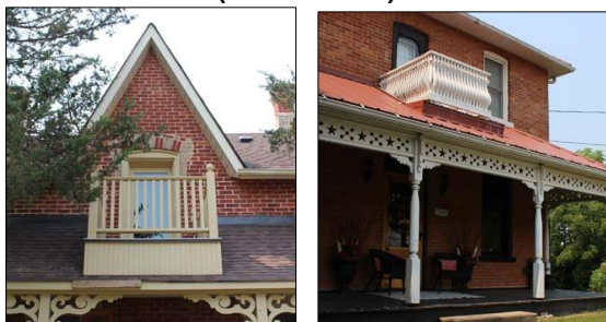
2864 County Rd. 27 & 70 Hearn St. – existing second floor balconies (Source: GDV)
