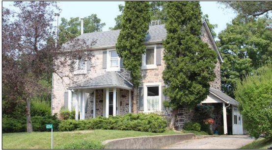
4354 Line 7 - Front entrance portico (Source : GDV)
