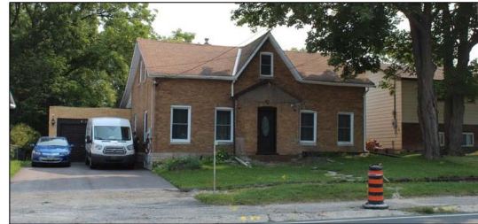
2887 County Rd. 27 – garage addition at rear of the property (Source: GDV)
