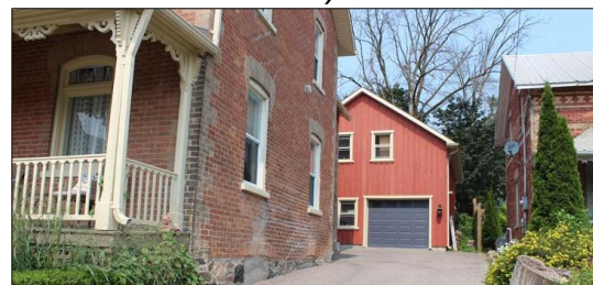
4334 County Rd. 88 – stand-alone garage structure located at the rear of the property (Source: GDV)
