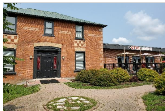
4240 County Rd. 88 – outdoor pathways (Source: GDV)
