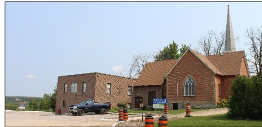
56 Hearn St. – Trinity Anglican Church Exposed stone foundation walls (Source: GDV)
