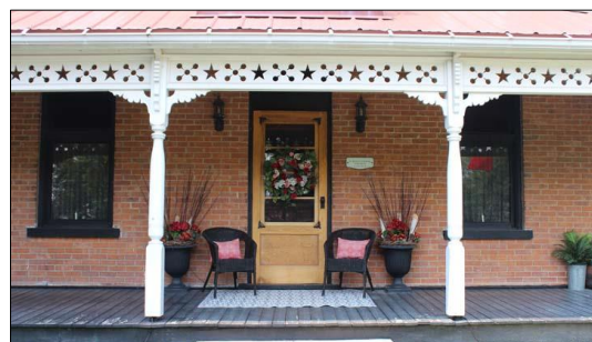
70 Hearn St. – Verandah (Source: GDV)
