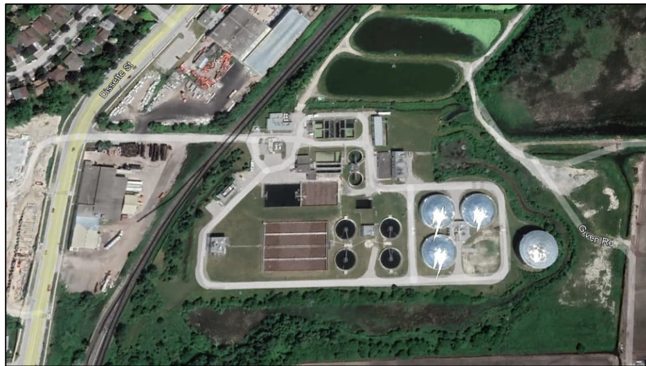
Figure 1-1: Aerial Photo of the Bradford WPCP (Google Earth, 2022)
