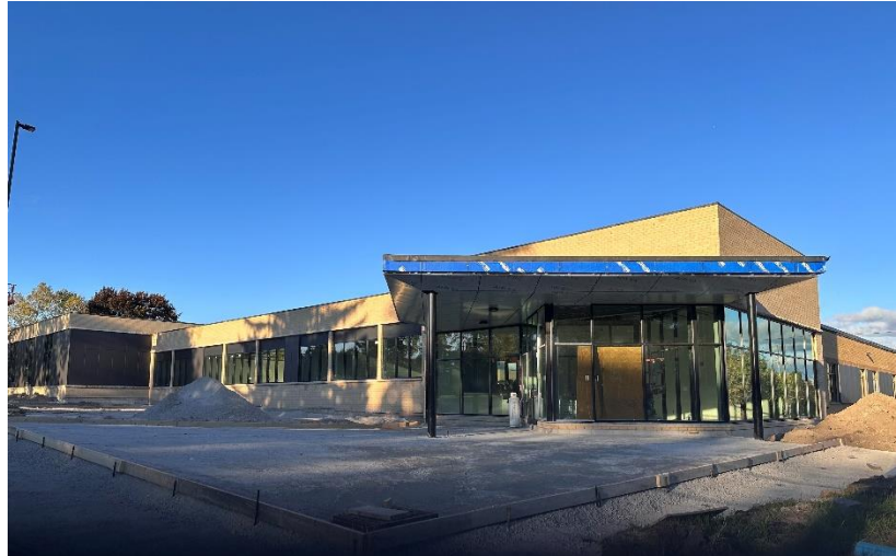
24: Exterior view of building at 177 Church Street
