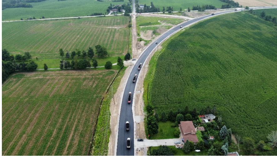
23: Aerial view of Sideroad 10, south to Line 5 during paving operations
